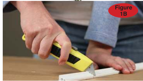
1B Cut Miracle Fit Base with a saw or knife to fit into the height size of window. (See figure 1A - from A to B)
