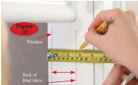
1C Measure from the window to the back of the roller blind fabric marking with a pencil in three different places top, middle and bottom. Draw a perpendicular connecting line and place Miracle Fit Base in alignment with the perpendicular connecting line.
