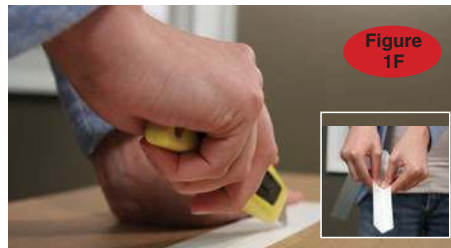
1F If necessary score and break away the Miracle Fit Extension to the desired width so that the gap between the wall and the blind is covered. Also cut the Miracle Fit extension to the desired height as shown in Figure 1A (from A-B).
