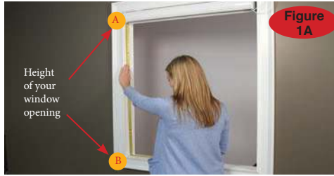
1A Measure the height of your window opening (A - B)
