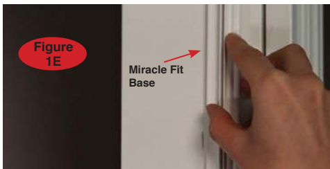
1E Press into place along the full height of the opening always following your perpendicular connecting lines which should be in line with the blind in the closed position.
